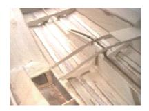
Cap with oversize ply, including a new centre section (it need not be "T" shaped as in the photo)
